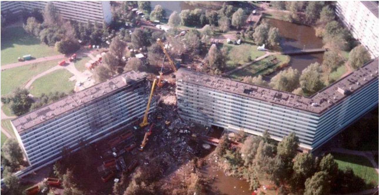
Figure 3 The Boeing 747 crash into high rise flats adjacent to Schiphol airport in 1992 [26]
