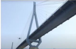
Port of Hamburg, used by HPA and HHLA, among others (crane inspection, site inspection, intralogistics, etc.)
