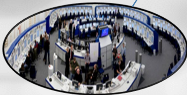
Automation and Connectivity
