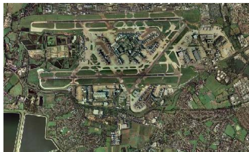
Figure 5: Heathrow airport (Source the Liaison Group of UK Airport Consultative Committees)
